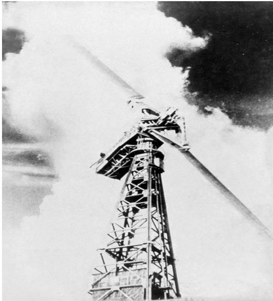
The world's first megawatt-sized wind turbine near Grandpa's Knob Summit,, Castleton, Vermont
