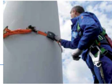
Fig. 3: Attaching a determined balance mass
