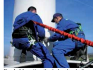
Fig. 1: Mounting the balancing belt
